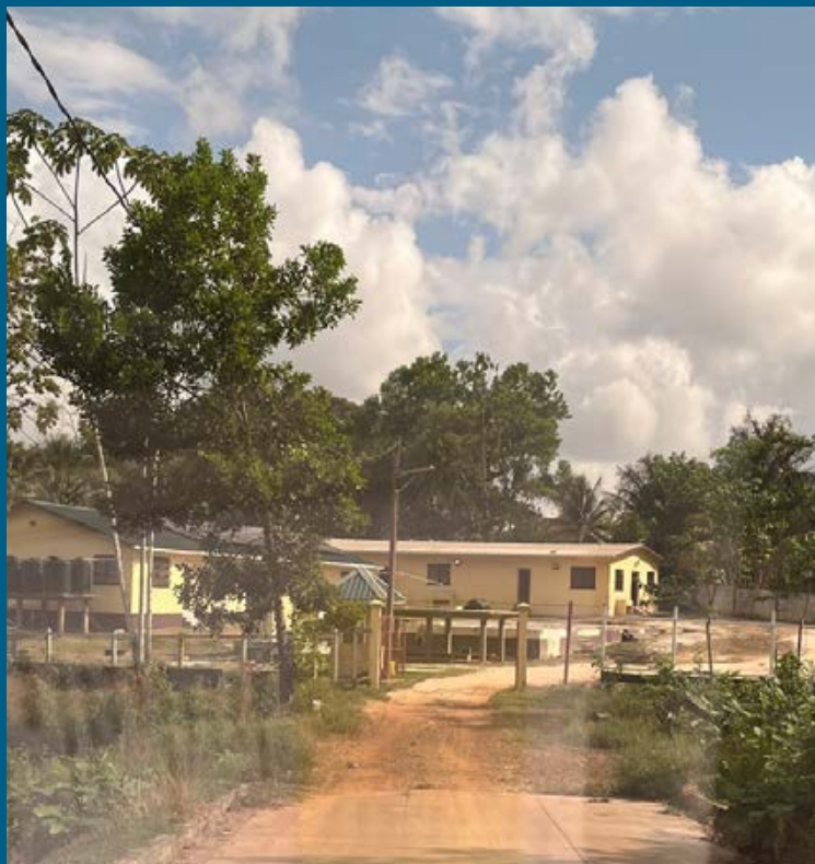
The Western Entrance to the dorm compound. Female Dorm's flooring is behind the Security Hut, male dorm on left and dining hall in background
